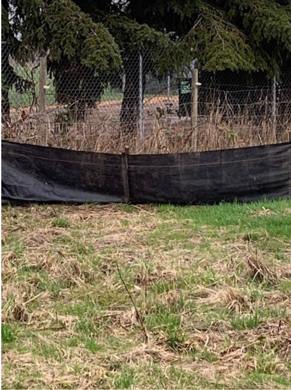
Erosion control measure on the alder St. three lot development.
